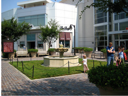
Figure 13 - Example of required public amenities: a fountain, plaza, and seating is used to satisfy the public amenity requirement
