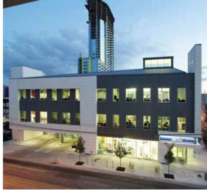
Figure 9 - Example of integrated parking structure: vehicular access is located at the rear of the building, with the garage façade and architecture matching that of the primary use
